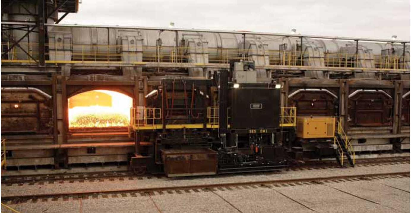
Fig. 20 Coke transfer car equipped with AP bearings
