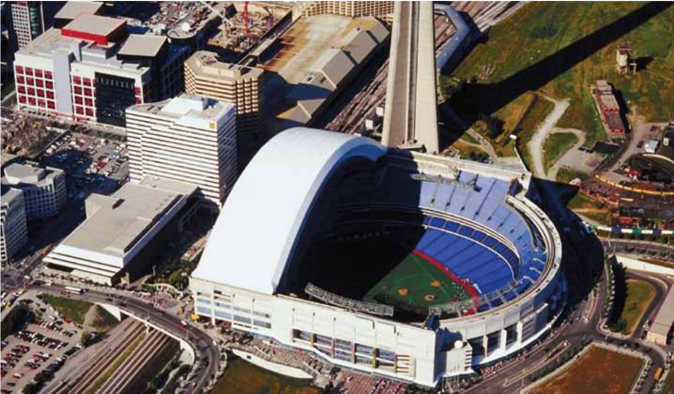
Fig. 7 The Toronto Blue Jays Stadium uses Timken bearings in the moveable stadium roof
